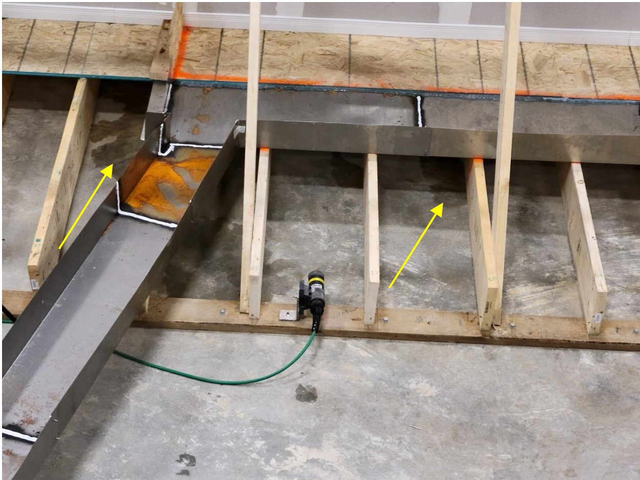
Figure 32. First evidence of leakage observed on top of the concrete pad in Phase 1 testing shortly after exposing the home to rising flood waters.
