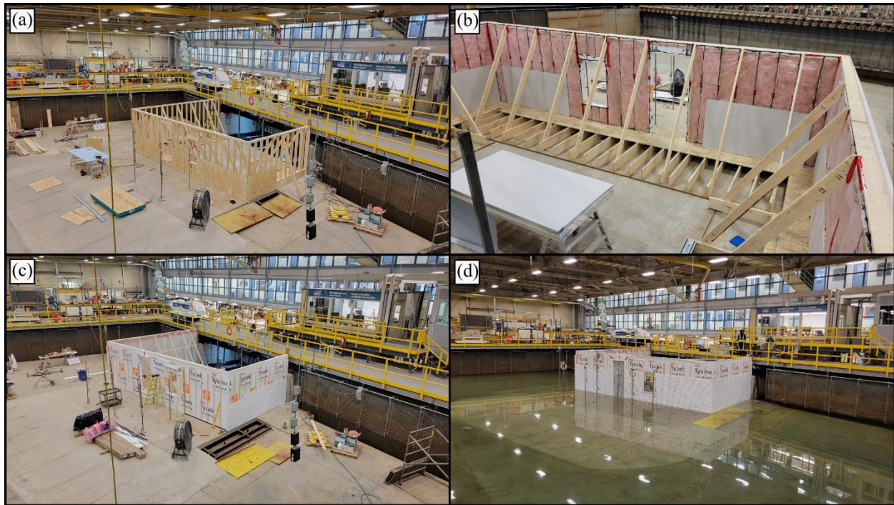
Figure 10. Construction of the Phase 1 superstructure. (a) Framing of superstructure; (b) superstructure with insulation and support structure installed; (c) superstructure with exterior cladding being installed; and (d) completed superstructure during testing.
