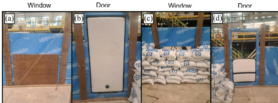
Figure 20. Opening barriers deployed in the MWB in Phase 2 – first set of tests: (a) plywood; (b) Flow Stop full-sized cushion; (c) sandbags; and (d) Flow Stop regular cushion.
